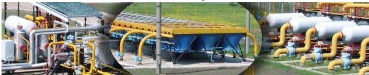
6. Gas coolers, gas driers and burning gas supply apparatus at the compressor station in Kursk. © LA
