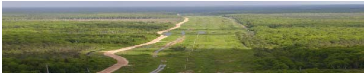
1. Route of the pipeline as seen from helicopter. The pipeline itself is 1.5 m under the ground © LA
