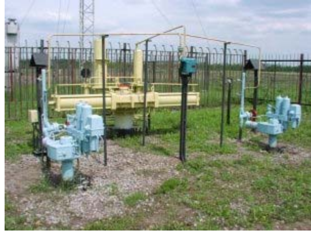
3. Valve node of the pipeline, which is under ground - near Kursk © LA
