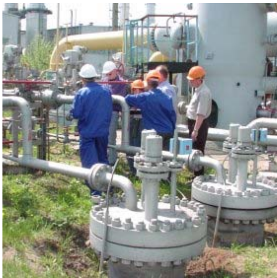
11. The team during measurements at the compressor station Davydovskaya. © LA
