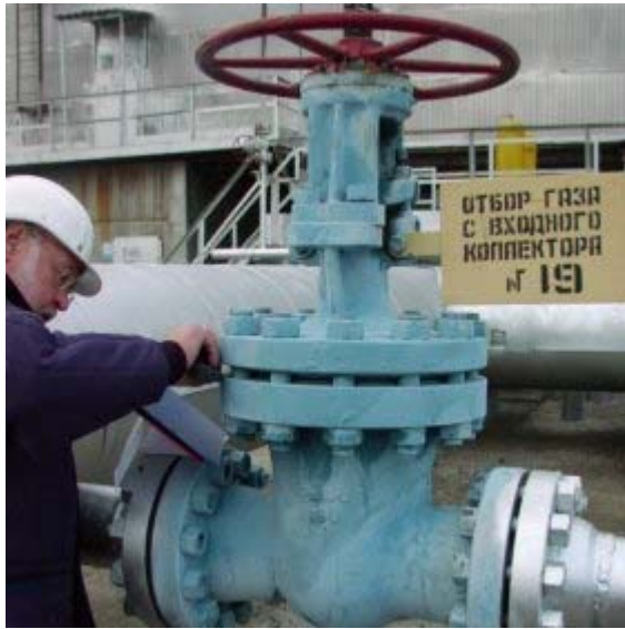
9. Screening of valve flanges © LA
