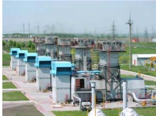
5. Compressors and turbines at the Kursk compressor station © LA
