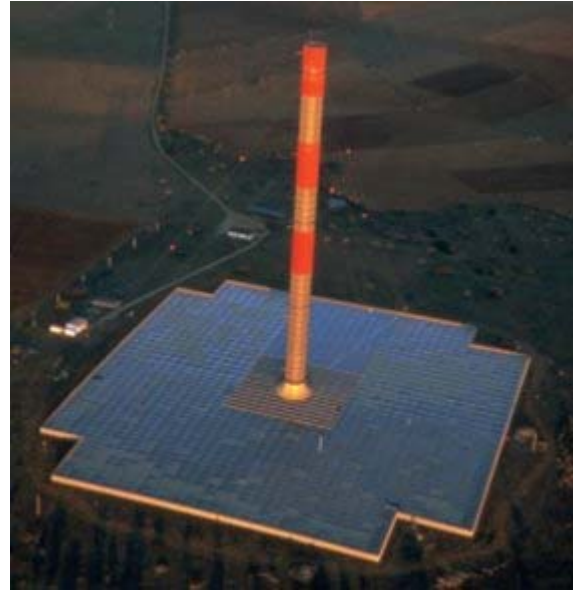
7. Solar thermal tower with an updraft wind turbine. Pilot project in Manzanares (Spain).
