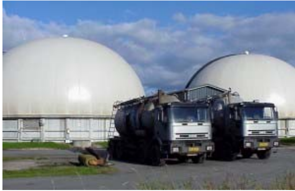
9. Bio gas storage © 2004 www.blaabjergbiogas.dk
