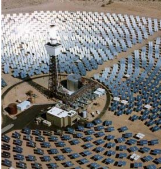
6. Solar thermal power plant at Barstow, California
