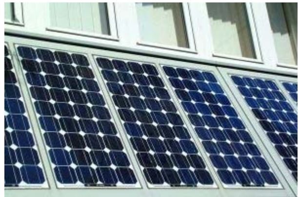
5. Solar cells as part of a house front © Freefoto.com
